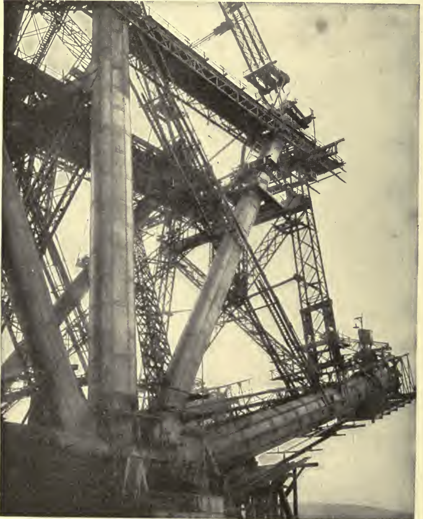
CONSTRUCTIONAL DETAIL OF THE FORTH BRIDGE Photo: Baker & Hurtzig
